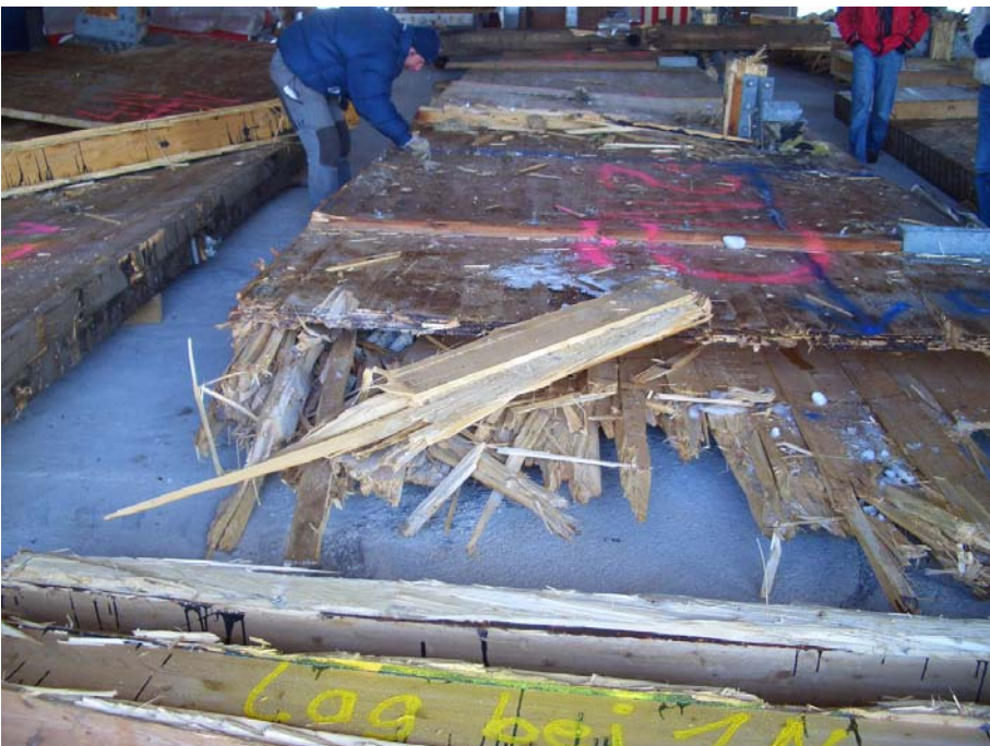
Figure 6 Damaged general finger joint of upper glulam girder due to water penetration (figure is presented upside down!)
